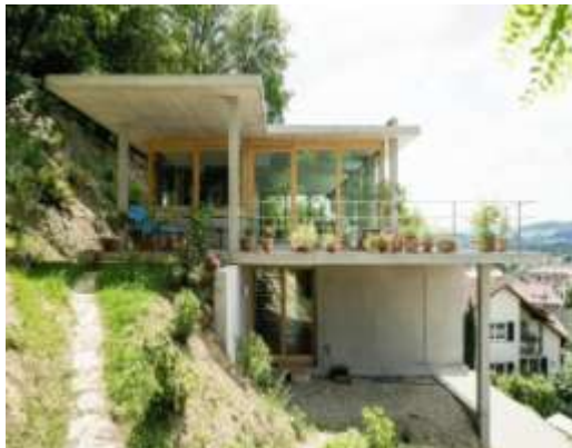
Figure 1 Actual Building located on slopy land
